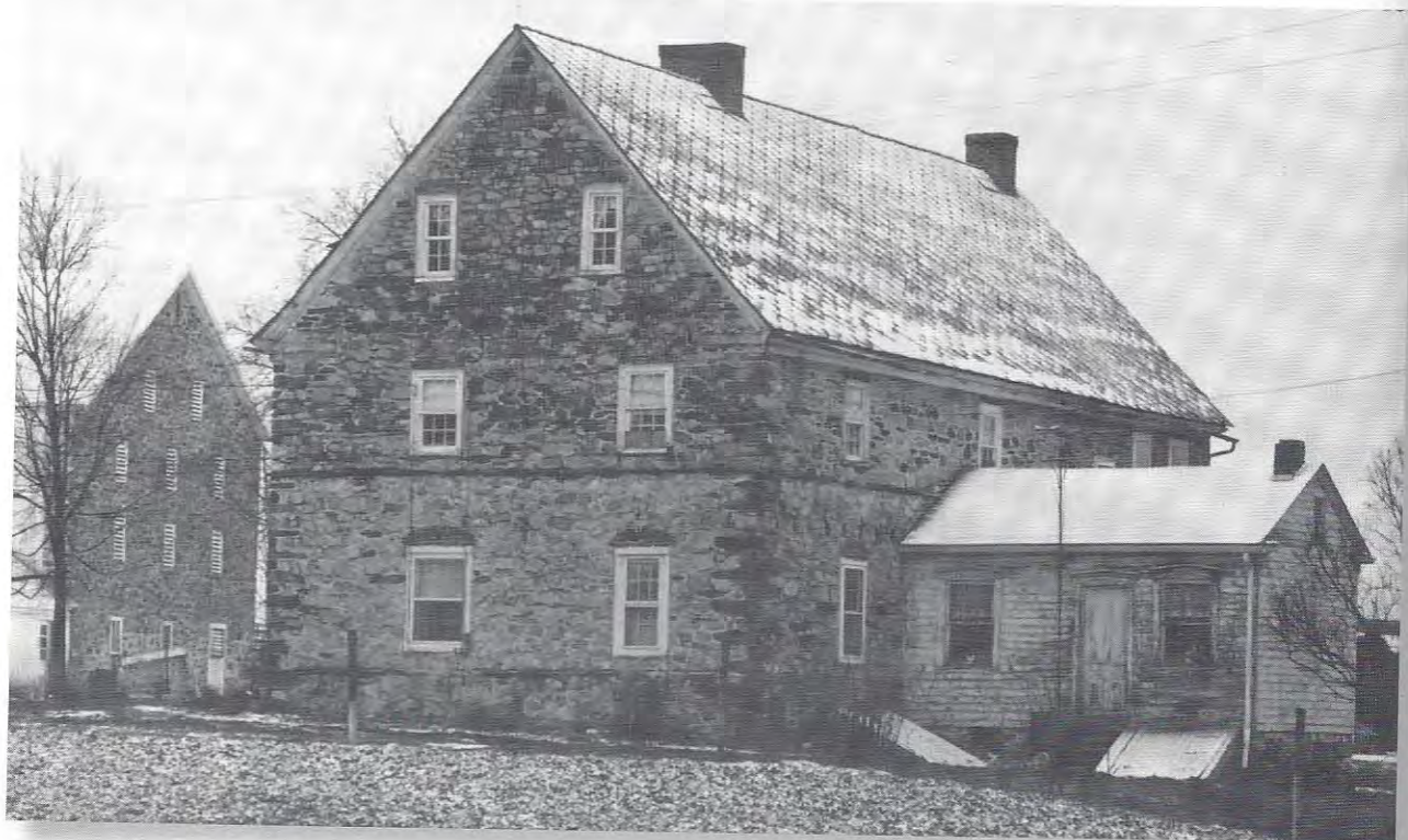
The Levans were French Huguenots who left Europe circa 1715. Abraham, one of four brothers, settled in the Oley Valley. The Abraham Levan Homestead, a medieval-style building, was erected in 1757. The massive stone walls and the very high-pitched roof give this house a character unique to the Valley. Note the brick arches over the windows. The house, located at 387 Bertolet Mill Road in Oley Township, is no longer in the Levan family. Courtesy of Oley Valley Heritage Association
